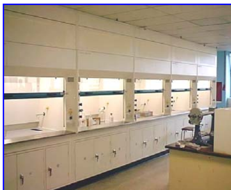
1500mm wide unit shown with infill panels and vented steel cupboards.
